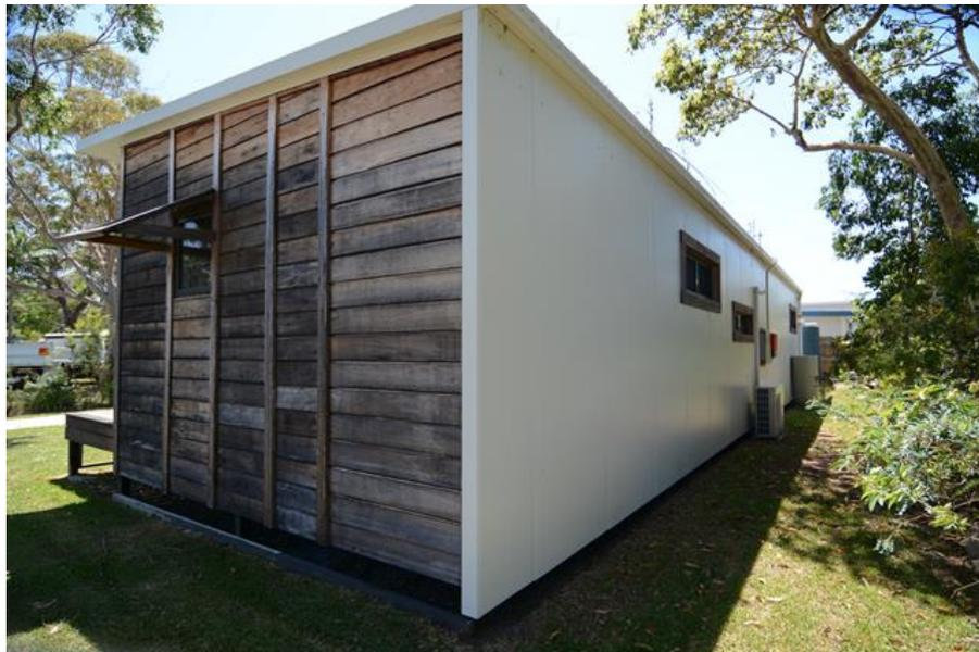
Figure 4b. Kingspan prototype house 1, showing the seamless integration of recycled materials and insulated panels, where the high thermal performance insulated panels are located on the rear wall (and the roof) to limit internal temperature rise on hot days.
