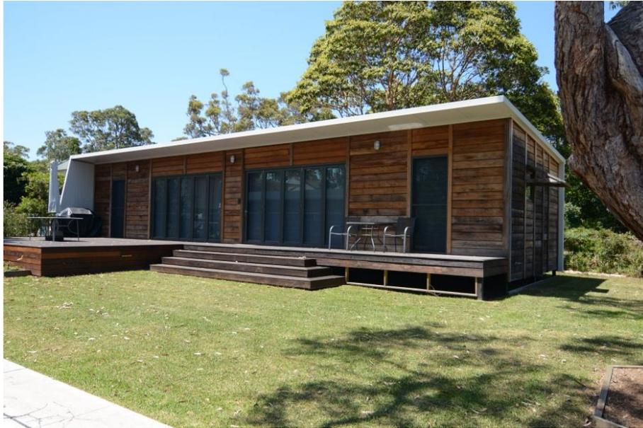
Figure 4a. Kingspan prototype house 1, with a shaded verandah which makes use of overhanging insulated roof panels. The front and side uses recycled hardwood to provide feature walling.
