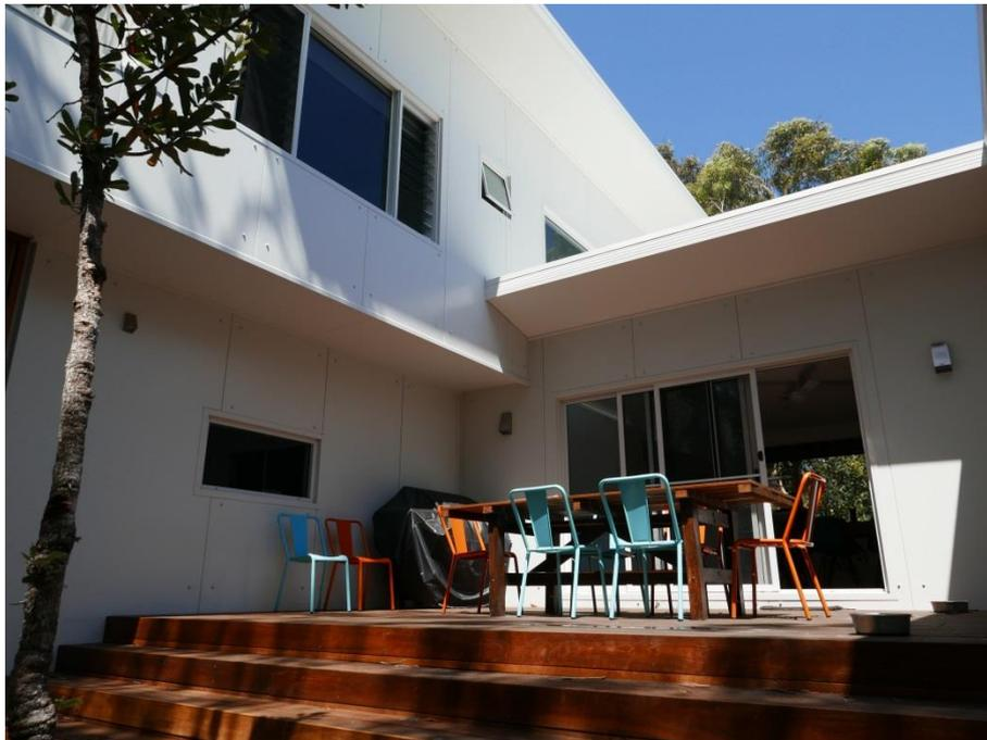
Figure 5b. Kingspan prototype house 2, showing good design versatility in the use of insulated panels. The high thermal performance envelope permits the opportunity for greater glassed areas, which is a feature of insulated panels typically used in retail shopping centre design to enhance design flexibility.
